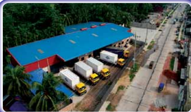
CNG Compressor Station at Bhola
