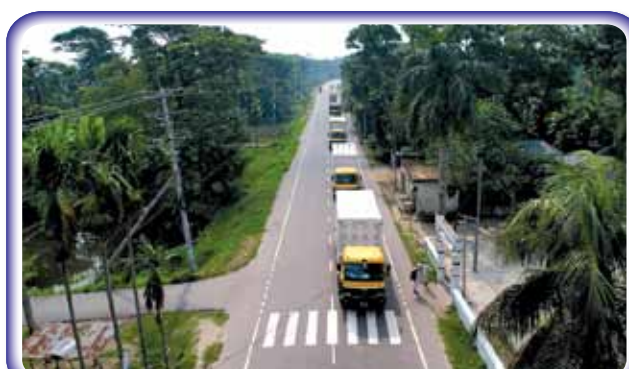
Cng Carriers Towards Different Industries
